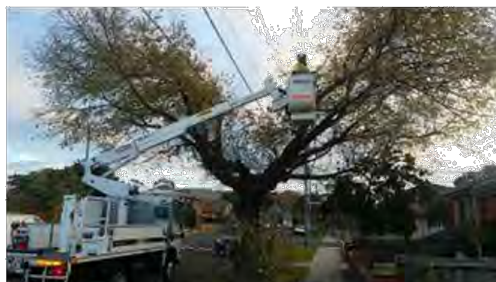
Street electrical line clearance works are generally undertaken by qualified Council Arborists in compliance with Electricity Safety (Electric Line Clearance) Regulations 2015 (see Table 22 for clearances)
